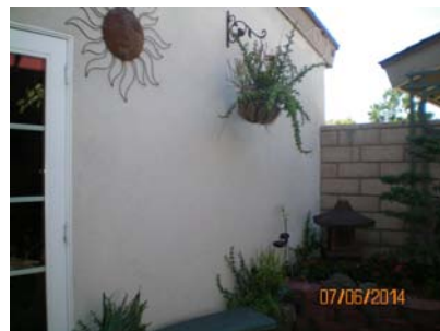
Wall before the transformation
